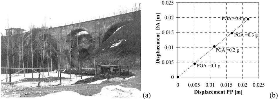
Figure 8: (a) Cevetta bridge; (b) correlation between the performance-point displacement (PP) and the maximum dynamic response (DA) - 1<sup>st</sup> mode force distribution.
