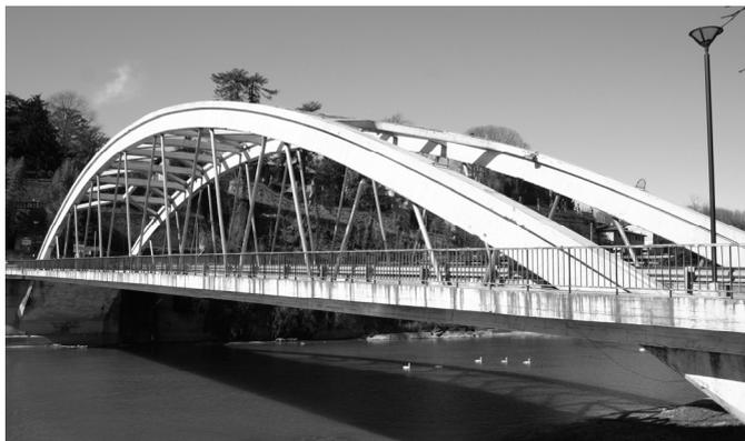
Figure 1 : View of the tied-arch bridge in Canonica d'Adda, Italy (1955).
