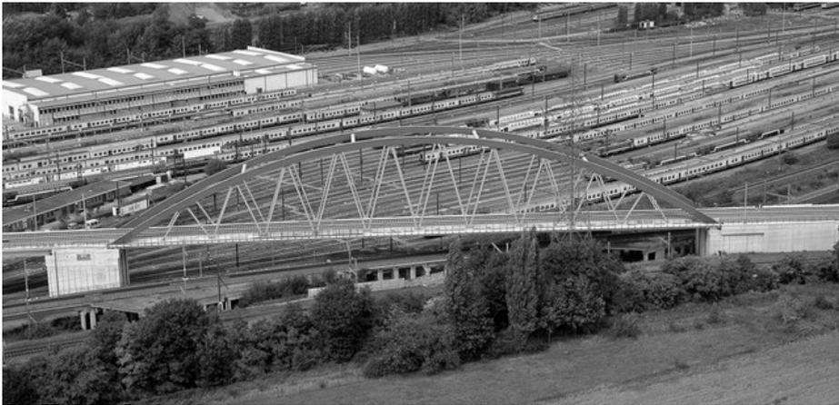
Figure 4 : Steel tied arch bridge Schaarbeek.
