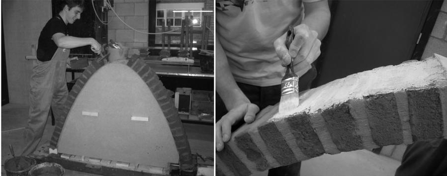
Figure 5: Construction of arch – limewashing of arch
