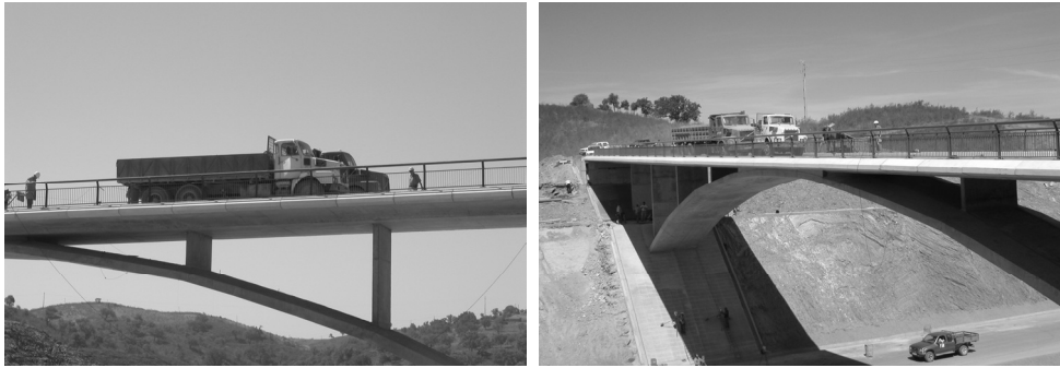
Figure 5 : Static load test
