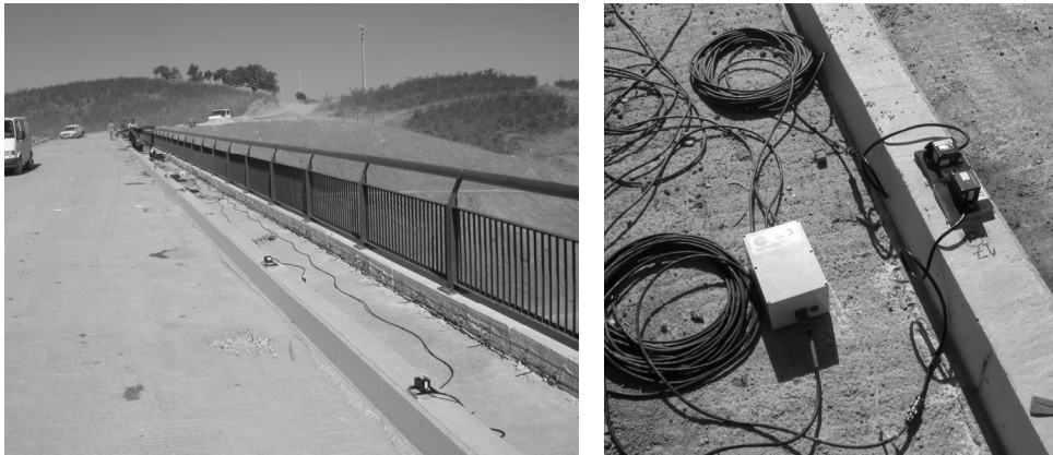
Figure 7 : Instrumentation during the dynamic tests
