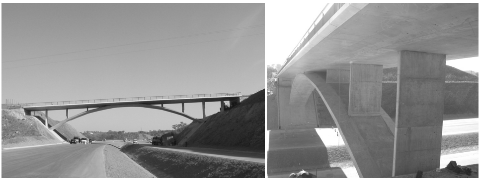
Figure 1 : The overpass bridge PS2
