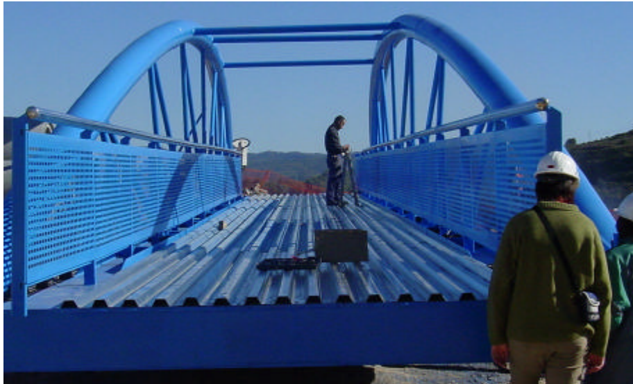
Picture 5: Inside before the launching
