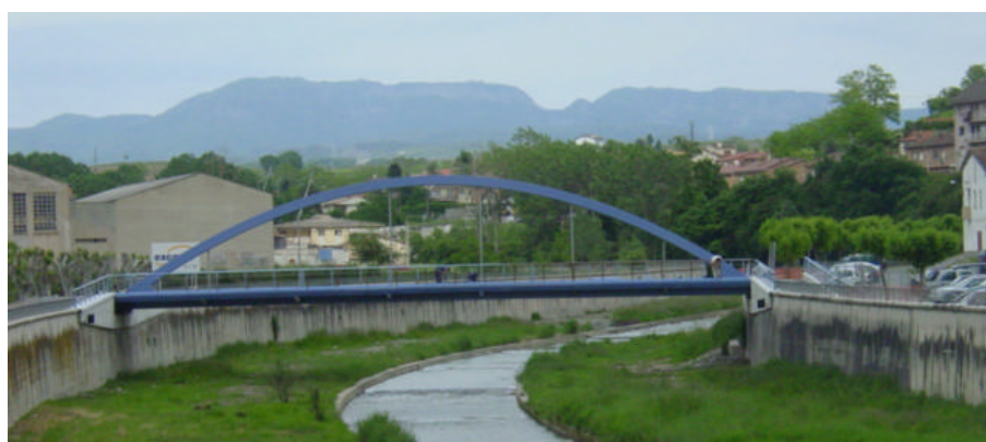
Picture 10: The footbridge finished
