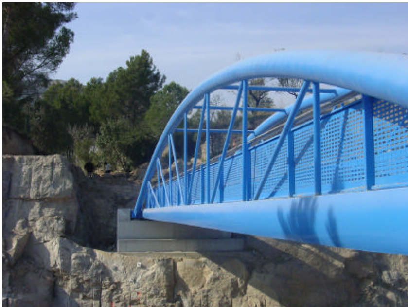
Picture 6: Side after launching
