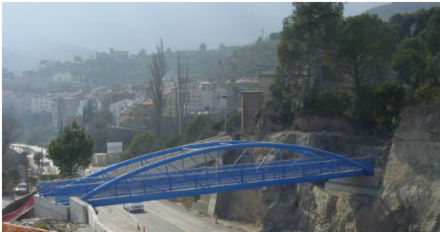
Picture 2: View of the Footbridge
