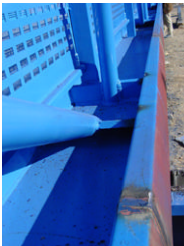
Pictures 3 and 4: Connection suspension cable-deck and arch-deck
