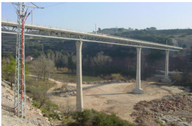
Picture 1: Bridge Puente del Centenario in Monistrol (Javier Manterola)
